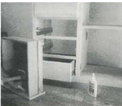
Attach drawer guides to boards Q and F. Nail the drawer fronts R and S to the drawer face panels using brads and glue.
