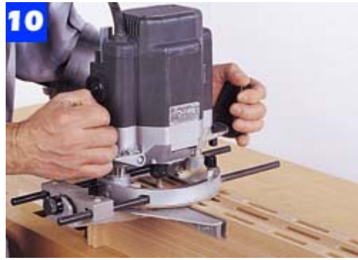
To cut the long row of mortises in each stile and rail, clamp three of the work-pieces together to support the router.
