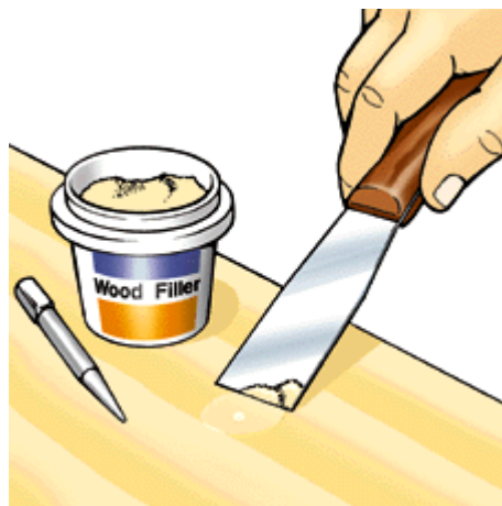
Fig. 11 Use a nail set to drive all nails below the surface. Then apply wood filler over the nailheads with a putty knife.
