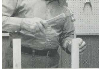
The frame sections of the china hutch are assembled with the aid of glue and spiral dowels. Dowel centers are recommended to ease matching of dowel holes.
