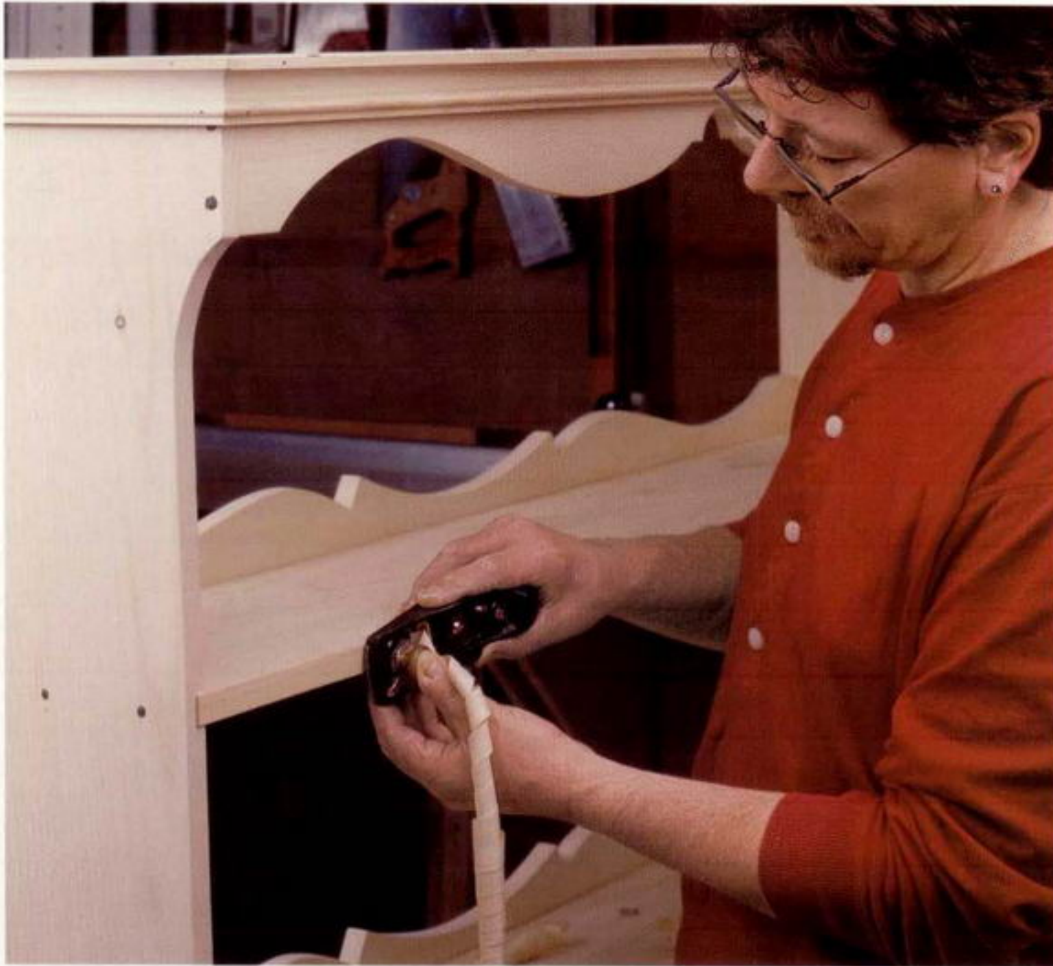
Photo 1: After installation, trim the front of each shelf flush with a sharp block plane.
